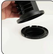
To do this, the existing diffuser is removed from the outlet. The existing diffuser can simply be pulled off with a little force.
